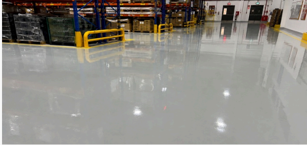
Industrial Epoxy Flooring
